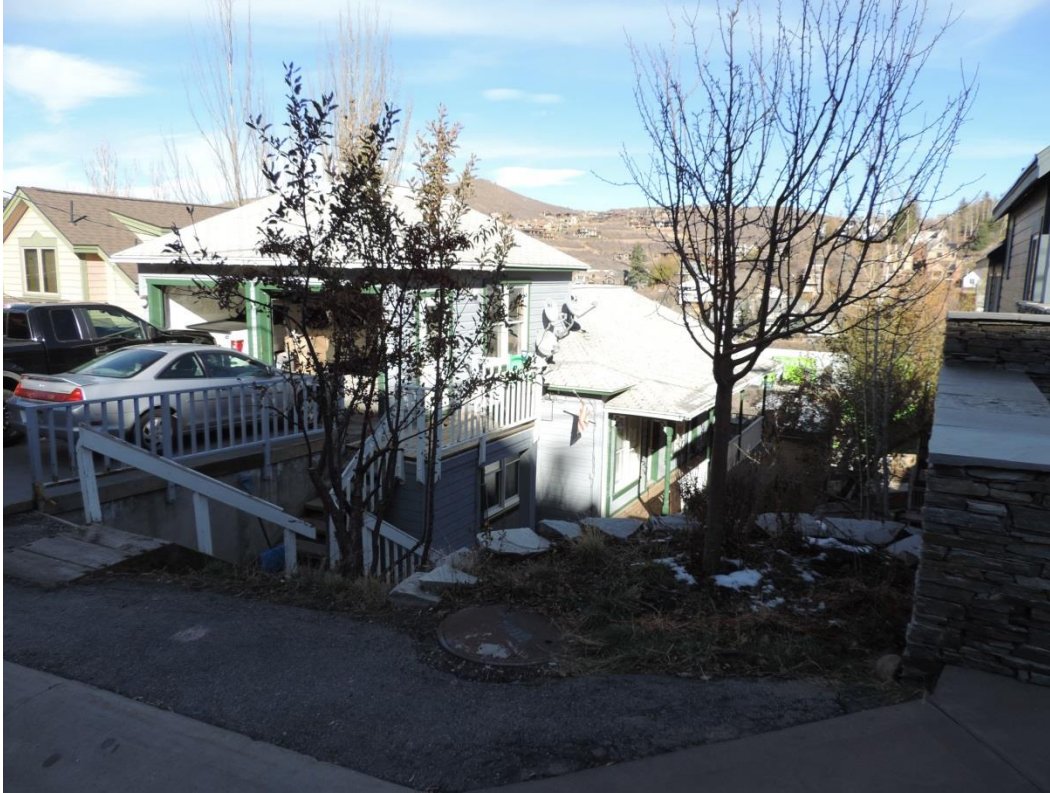
Photo No. 2: Northwest oblique. Camera facing southeast. November 2014.
