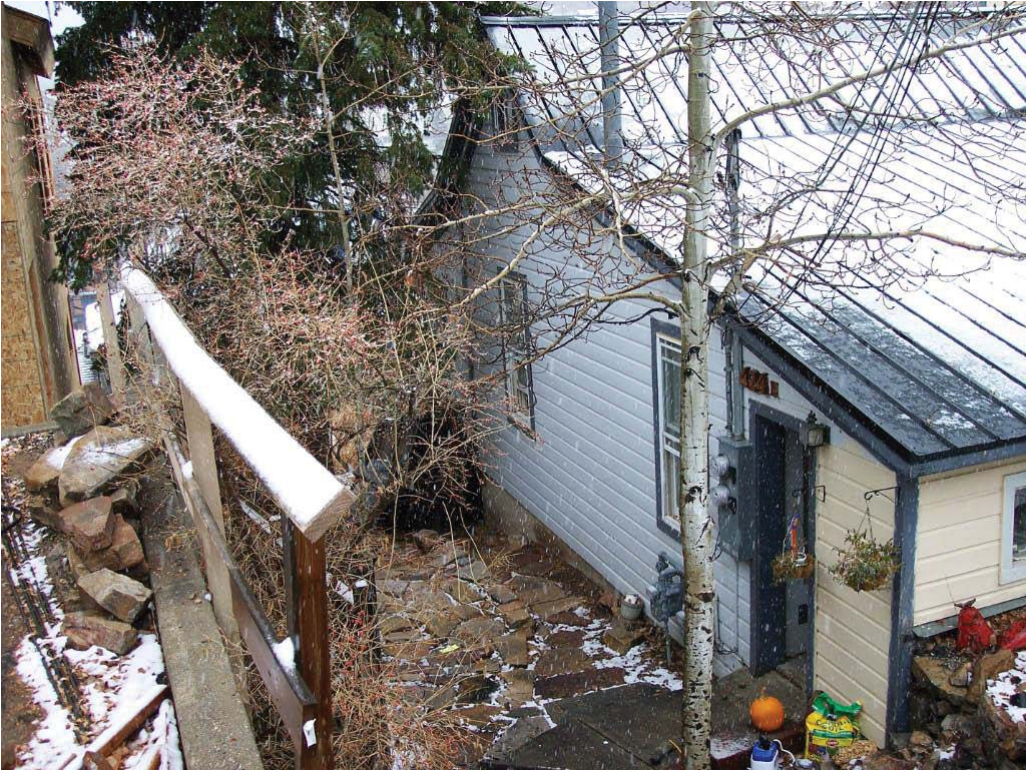
Stone walkway at entry leading to rear yard (north elevation)
