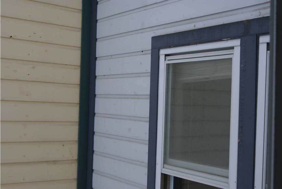
Typical exterior trim
