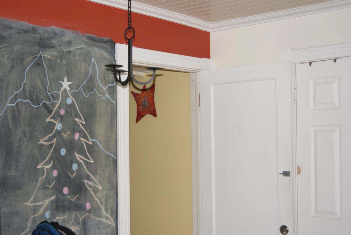
Typical ceiling trim and door casing
