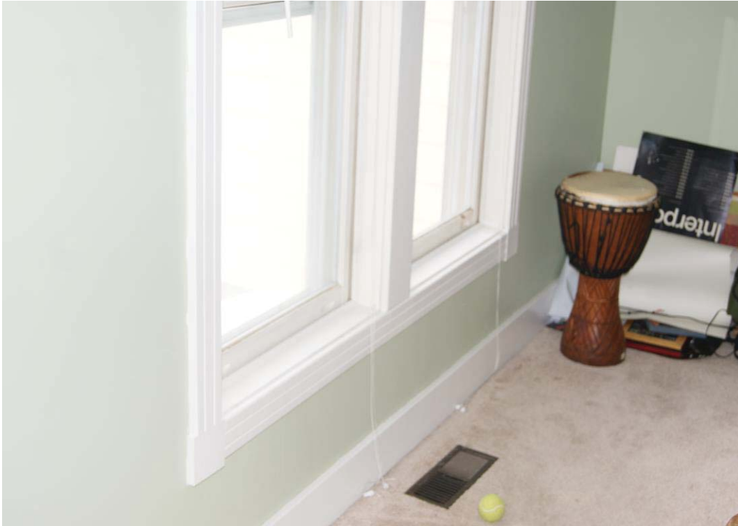
Typical base and window casing
