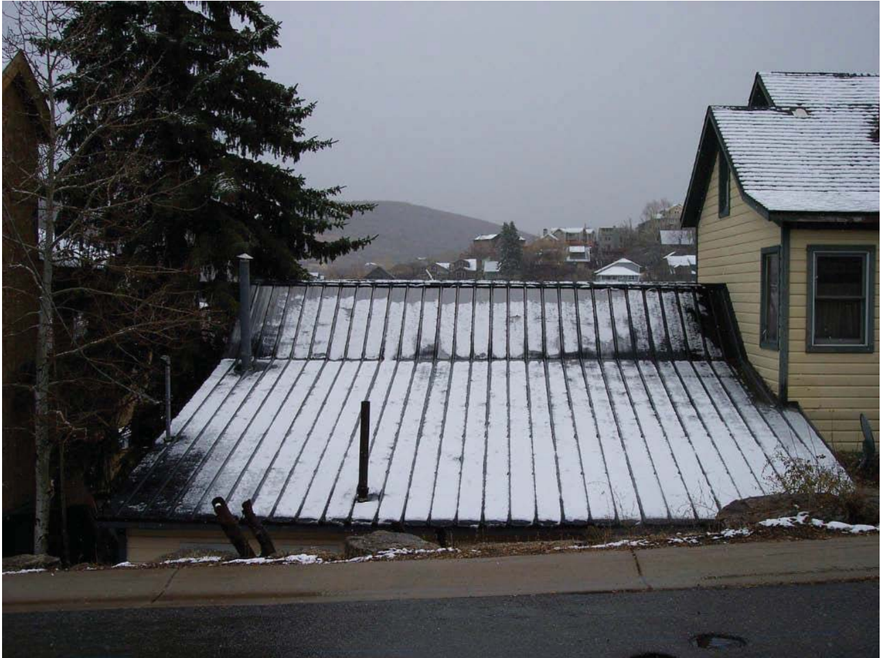
Roof looking east
