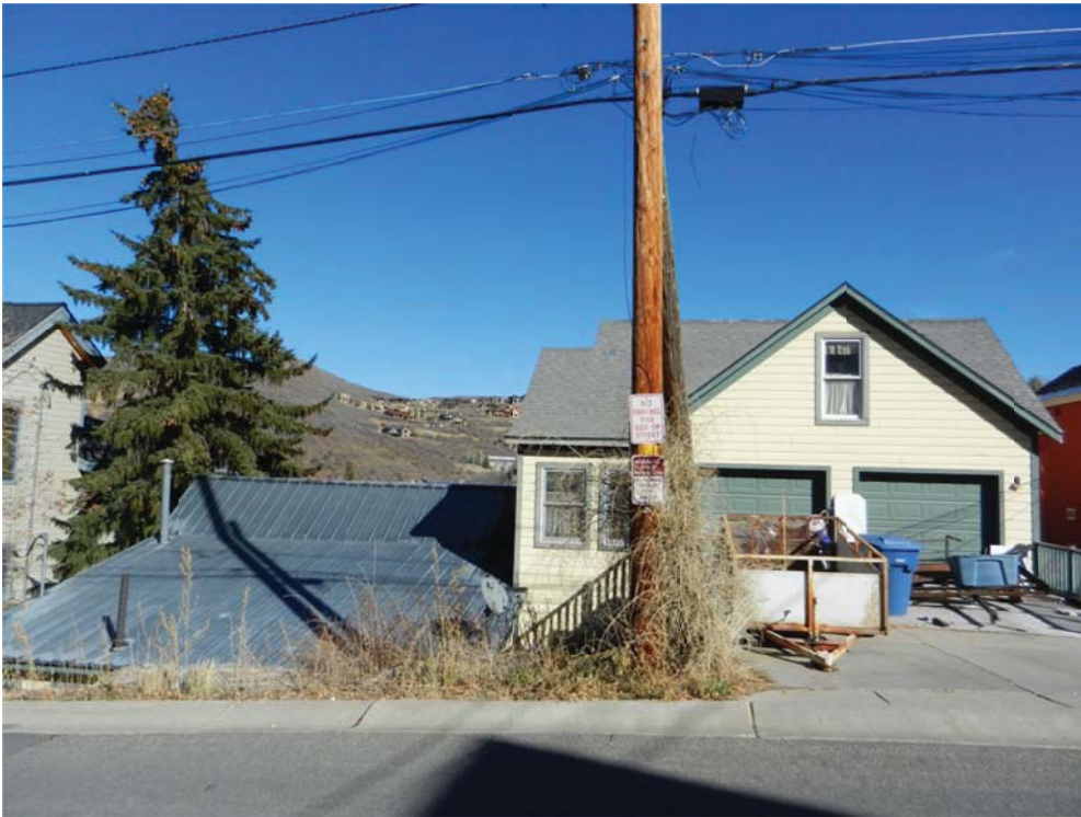
424 Woodside Avenue. West elevation. November 2013.
