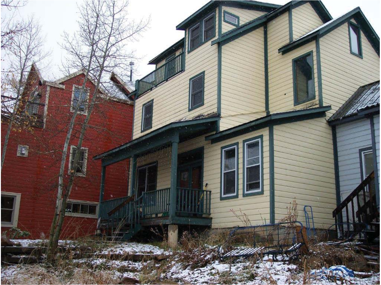
Addition on the south elevation built after 1993
