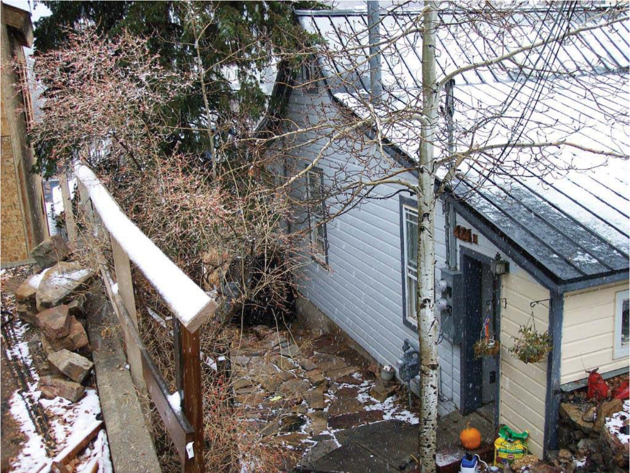
Roof looking southeast
