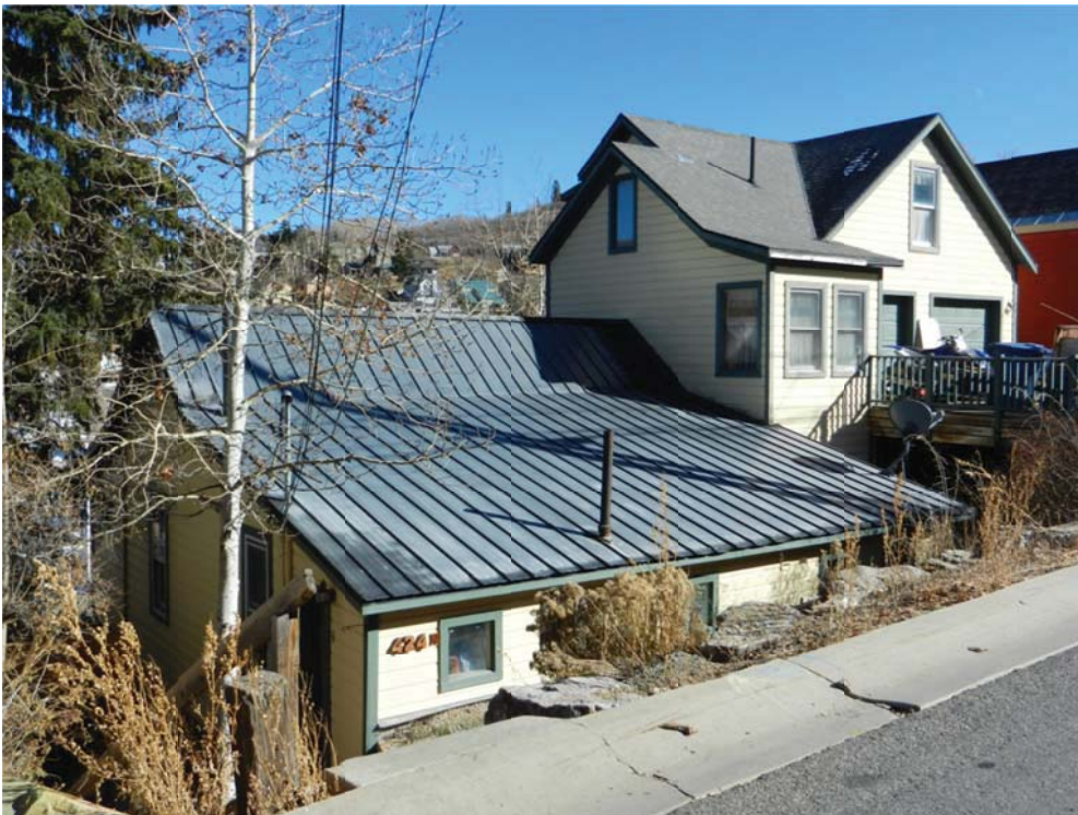
424 Woodside Avenue. Northwest oblique. November 2013.
