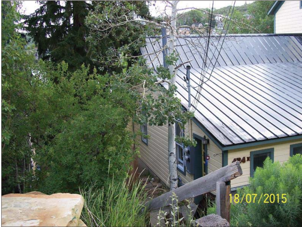
Figure 6. North and west sides of historic house at 424 Woodside, facing east-southeast, 2015.
