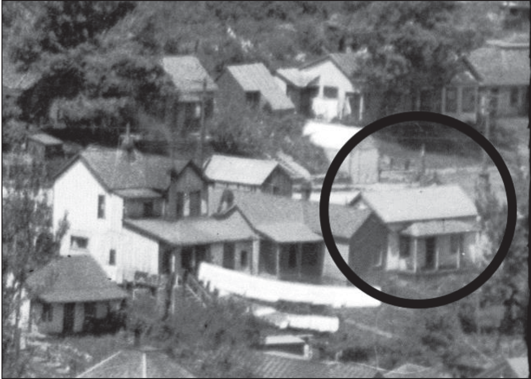
Figure 4. View of property at 424 Woodside in 1930, facing northwest. Note the retention of the simple hall-parlor form and addition of hip-roofed front porch, which was removed by 1941 according to the Sanborn map. Photograph no. 1987-2-134.
