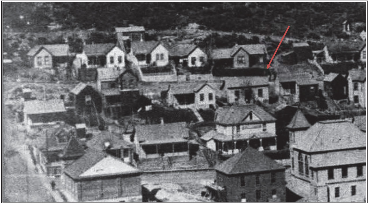
Figure 3. View of property at 424 Woodside in 1907, facing west-northwest. Note simple hall-parlor form, east-facing aspect with a view across canyon, and access via a footpath leading north from Fourth Street behind the Park Avenue houses. Note the absence of a front porch on east side, although according to the 1907 Sanborn map a porch was added in this year. Also note the mix of house orientations along the downhill (east) side of Woodside, with some facing the street and others the canyon. Photograph provided by Jonathan DeGray.
