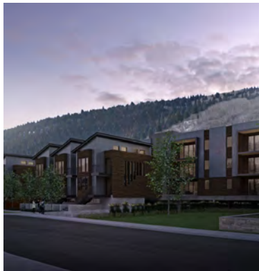
WOODSIDE II* PARK CITY, UT
